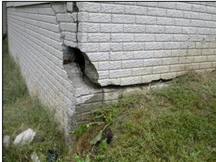
3. Failed foundation
