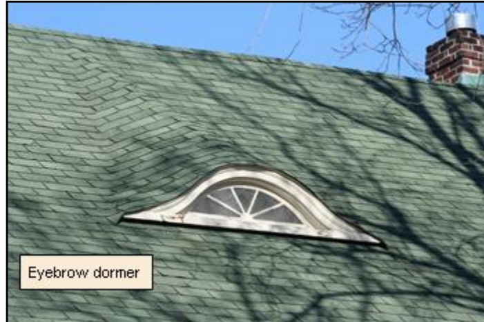
1. Asphalt roofing with decorative dormer
